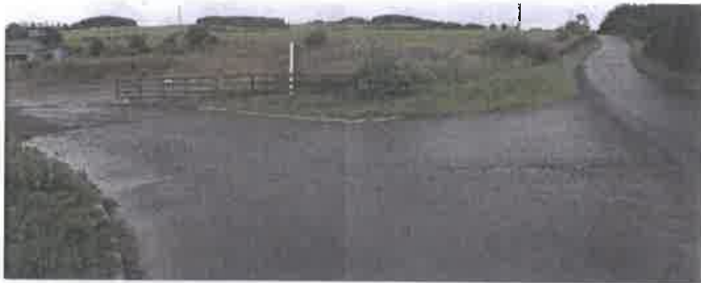
Figure 6. The existing site entrance
